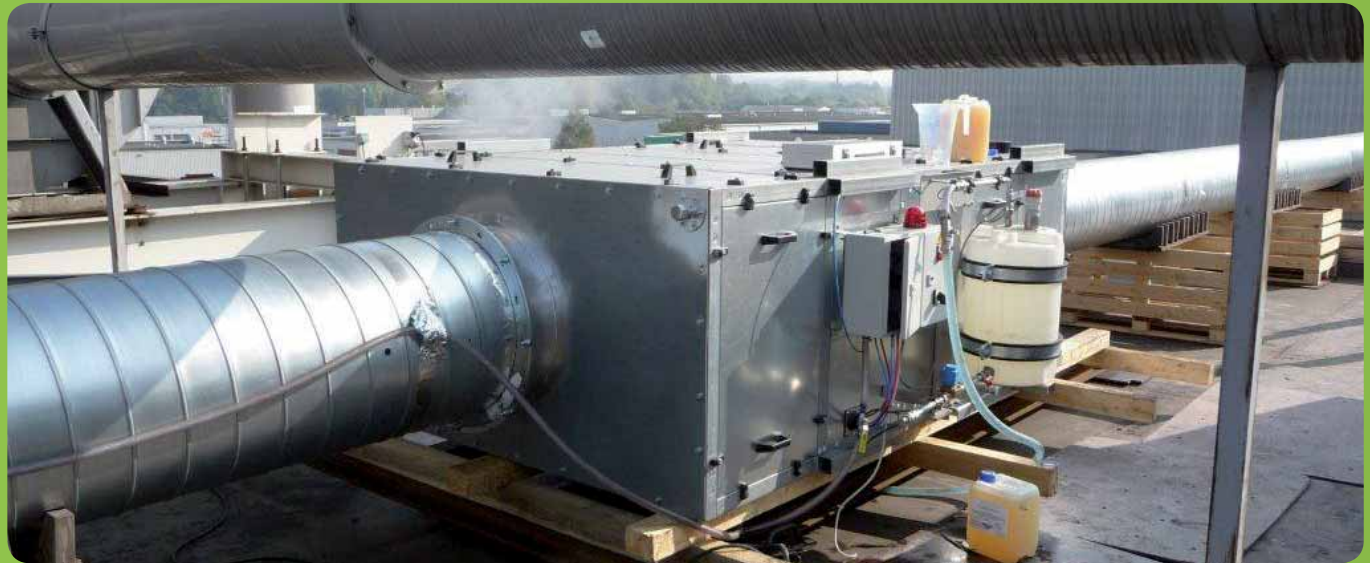
Test installation on the roof of Componenta Heerlen foundry; reaction chamber with tank for aqueous solution of essential oils.
